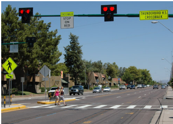
Typical installation of Pedestrian Hybrid Beacon
