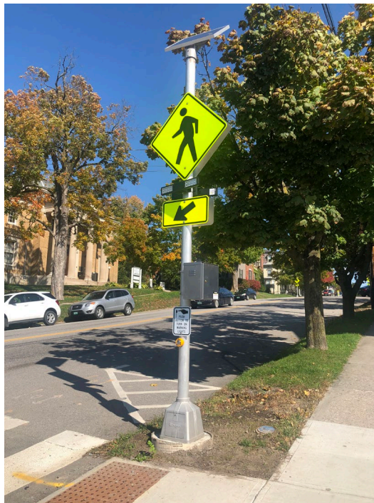
Photo of RRFB installation at a marked crosswalk.
