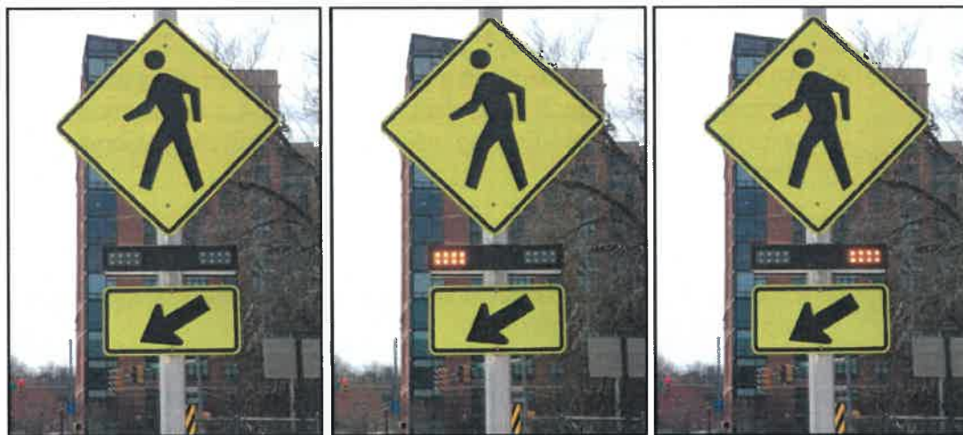
Figure 1. Example of an RRFB dark (left) and illuminated during the flash period (center and right) mounted with W11-2 sign and W16-7P plaque at an uncontrolled marked crosswalk.
