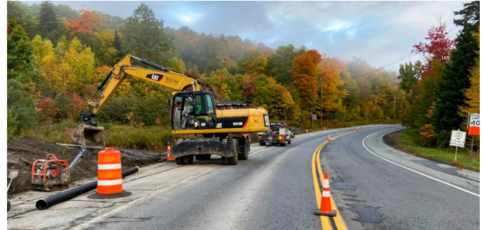
WILMINGTON - BRATTLEBORO. In 2021, a multi-year road reclamation project began along VT Route 9. By 2023, this 12.5 mile stretch of highway will feature new pavement, culverts, guardrail, and other safety improvements.
