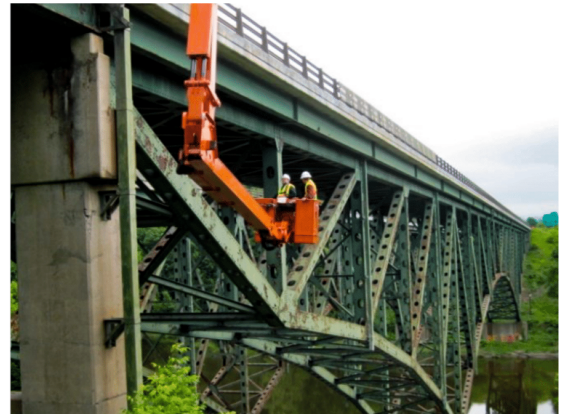
STATEWIDE. Bridge Inspection Crews are busy throughout the year, getting to those hard-to-reach places to accurately assess structure conditions.
