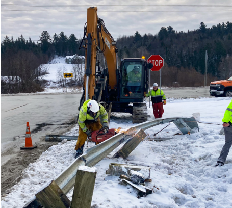
Winter maintenance is about more than just snow plowing. Despite the cold temperatures, VTrans crews spend a good portion of the winter months repairing and replacing damaged guardrails to keep the roadway safe for motorists.
