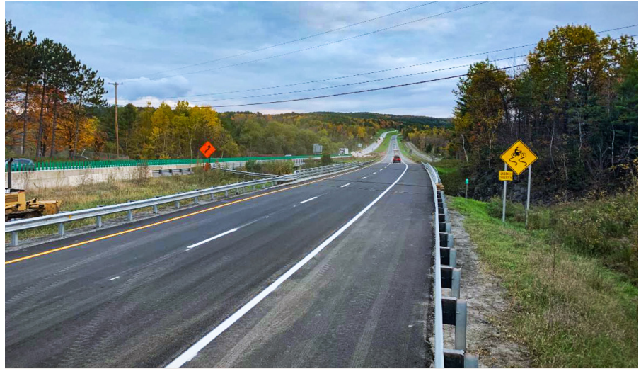
BERLIN. 2021 brought the completion of the I-89 Berlin bridges project, fully replacing the bridge decks for southbound and northbound traffic over VT Route 62 and Crosstown Road. Crossover traffic patterns were used during construction to allow traffic to flow in both directions while different bridges were closed for work.
