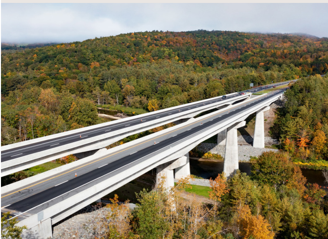
ROCKINGHAM. The new bridges along I-91 spanning the Williams River feature a unique construction method utilizing pre-cast concrete. These pre-cast concrete girders weighed almost 93 tons each.
