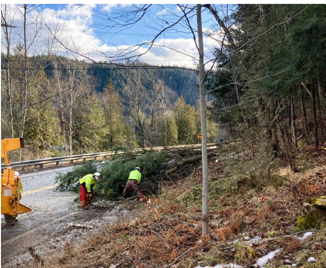
GREENSBORO. Highway maintenance often involves activities off the roadway itself. Our crews stay busy throughout the year cutting back vegetation to help with sight distances and improve safety in the area.
