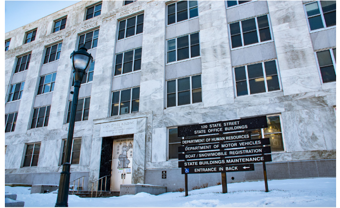
MONTPELIER. 120 State Street located directly across from the Vermont State House has long served as DMV headquarters.
