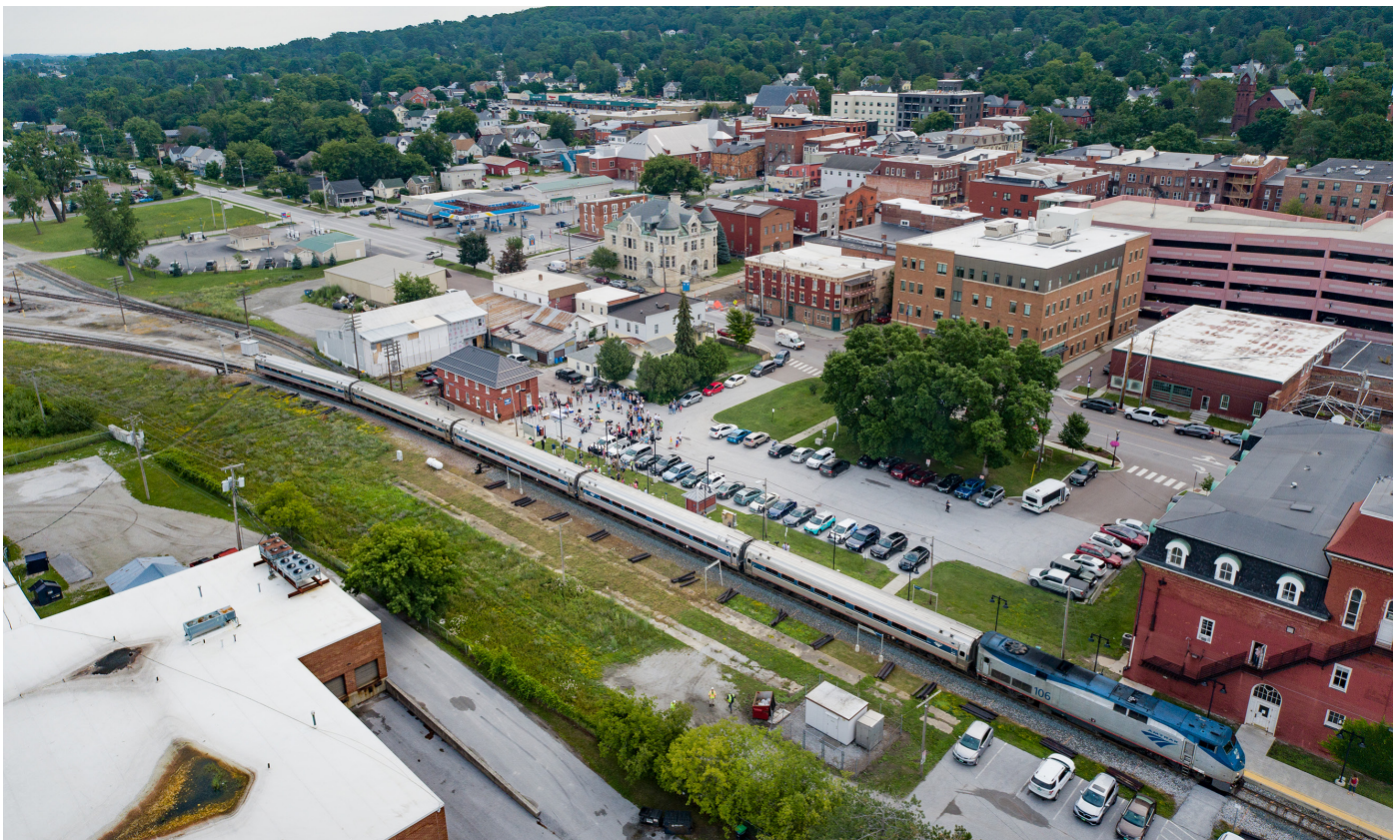
ST. ALBANS. The return of Amtrak services in mid-July 2021 was kicked off with a "Welcome Back" event at St. Albans Station. Officials from federal, state, and local government joined with excited rail enthusiasts to take the inaugural ride from St. Albans to Essex Junction.
