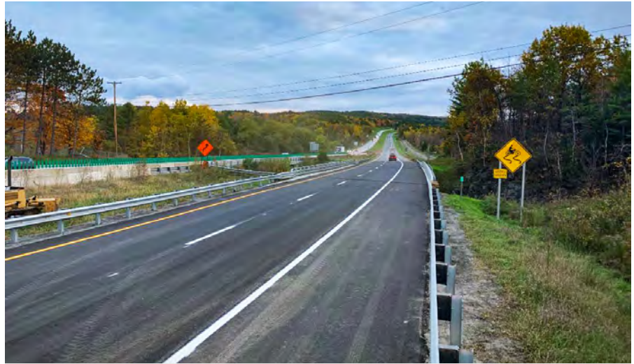
BERLIN. 2021 brought the completion of the I-89 Berlin bridges project, fully replacing the bridge decks for southbound and northbound traffic over VT Route 62 and Crosstown Road. Crossover traffic patterns were used during construction to allow traffic to flow in both directions while different bridges were closed for work.
