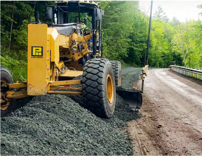
CAVENDISH-WEATHERSFIELD. 2021 marked the completion of a full depth reclamation of VT Route 131, including improvements to areas along the route that had substantial damage from Hurricane Irene.
