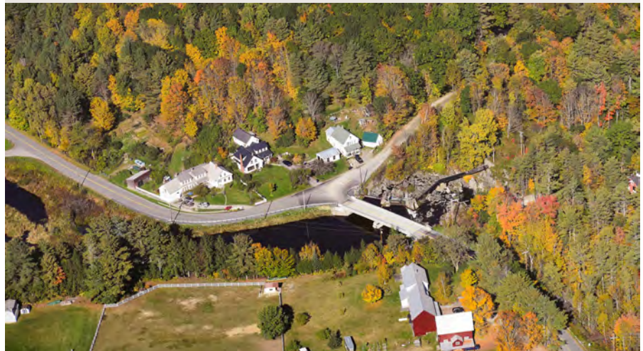
NEWBURY. The Boltonville Bridge over the Wells River connecting US Route 302 and Boltonville Road received a major face lift this past season as crews fully replaced the bridge deck and steel beams. New bridge joints were also installed, along with minor repair work to the concrete substructure. These improvements will increase the longevity of the bridge and will protect the structure from further deterioration due to chlorides.
