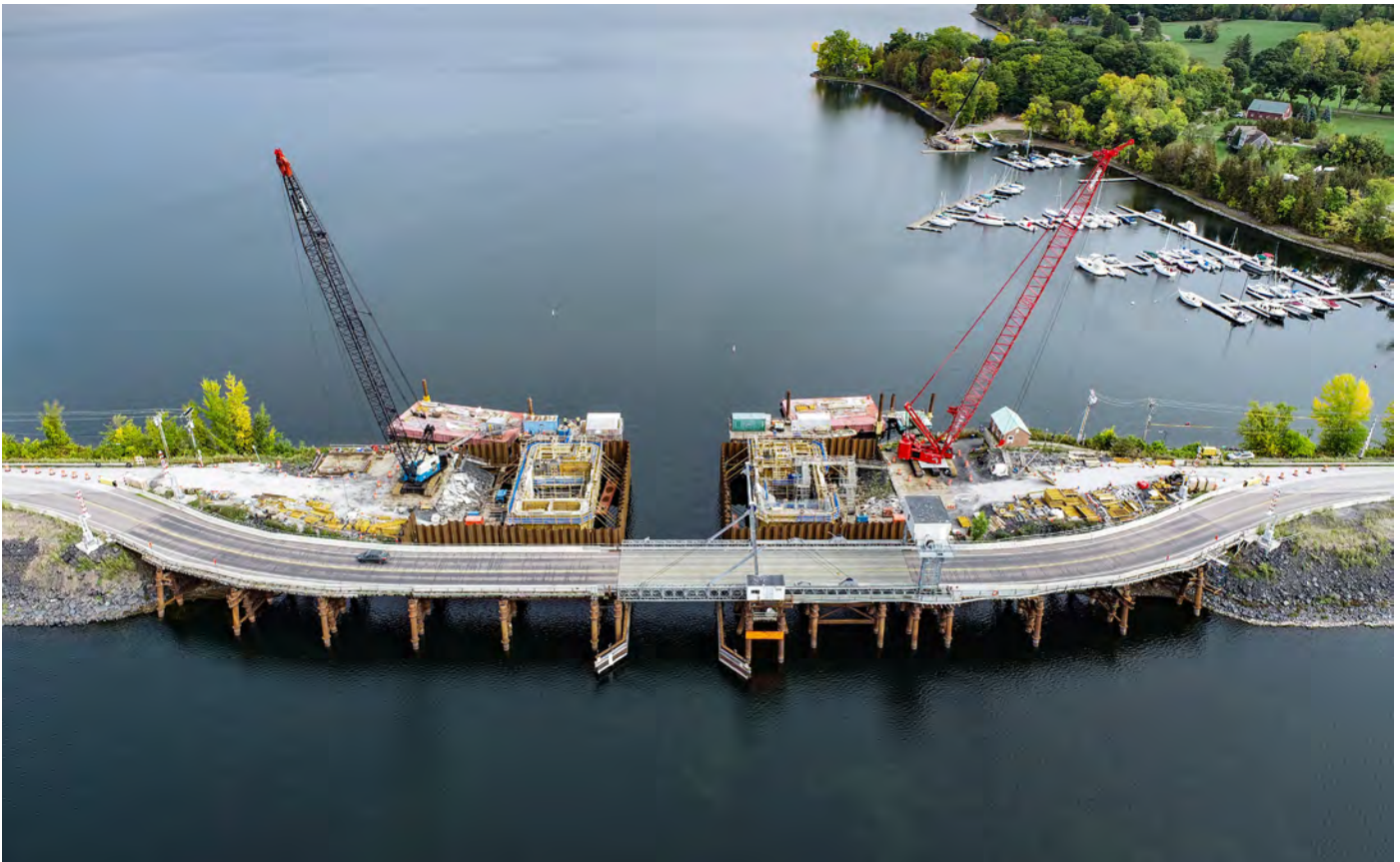
NORTH HERO - GRAND ISLE. The past year brought another busy season of construction on the US Route 2 Drawbridge replacement project. The structural concrete for the new bascule piers was completed as crews began erecting steel and preparing for the installation of the new drawbridge control house.
