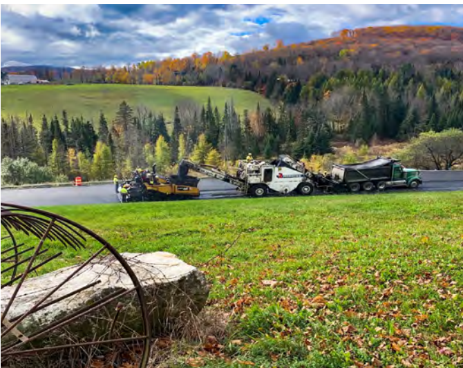
CHELSEA-THETFORD. A 15-mile stretch of VT Route 113 is under a full depth reclamation project. The original roadway was stripped to gravel and then rebuilt, along with ditching, guardrail, and alignment improvements. Paving of the final course is planned for 2022.
