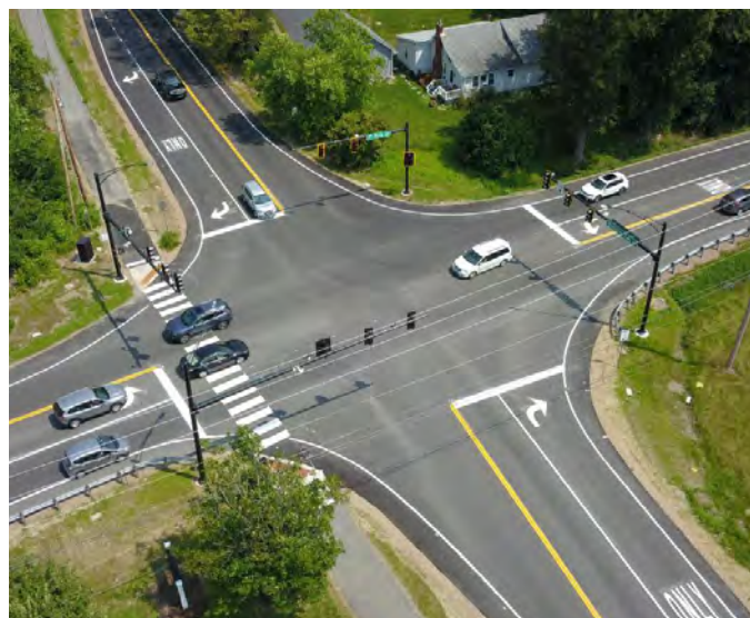
HINESBURG. An intersection improvement project was completed along VT Route 116. Improvements include a widened roadway, new turn lanes, and a new traffic light system to make the flow of traffic safer and more efficient.
