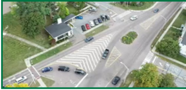
Existing aerial view of rotary
