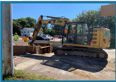
Crews excavating for waterline installation (l) and mechanical hammering to remove ledge (r).
