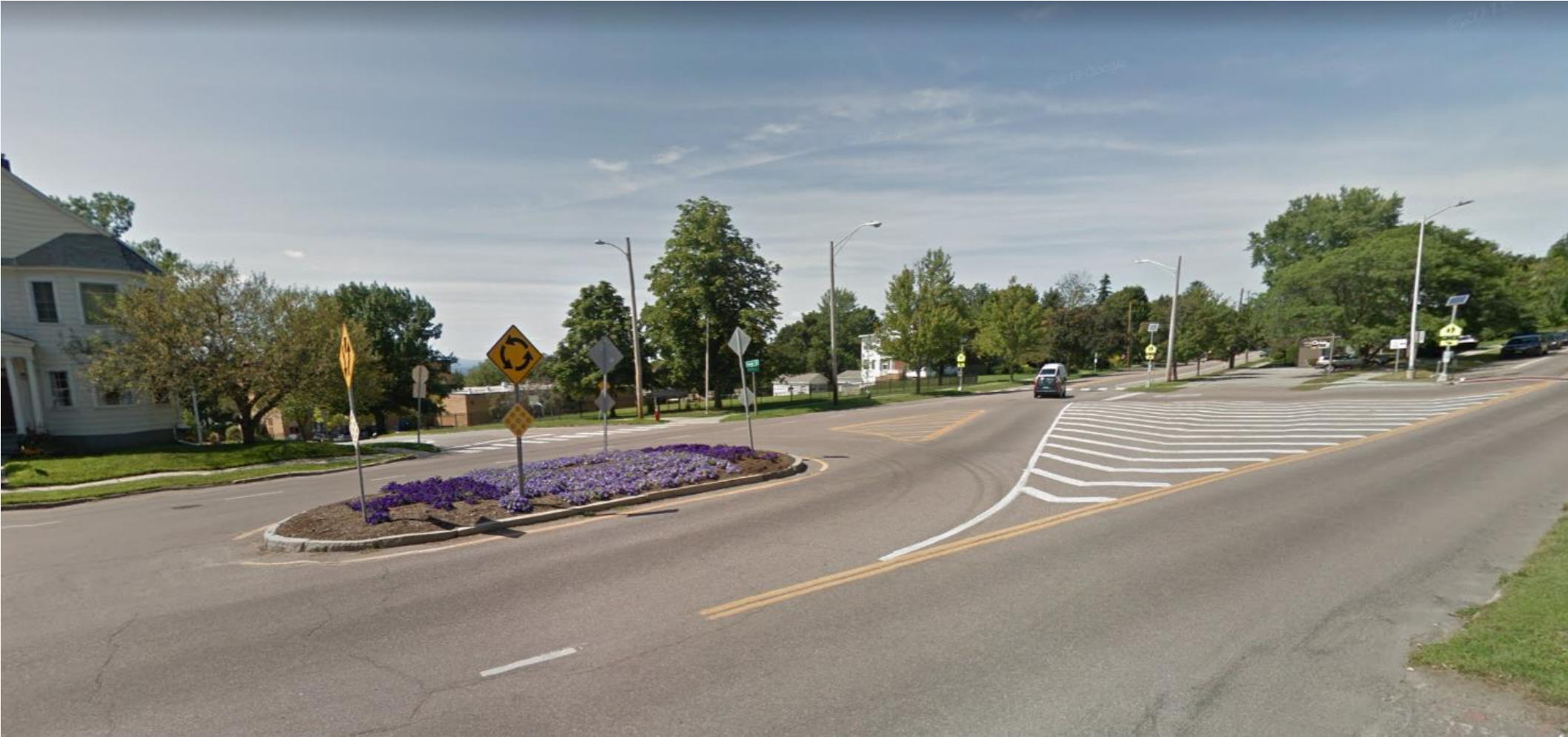
Shelburne Street Roundabout Project
