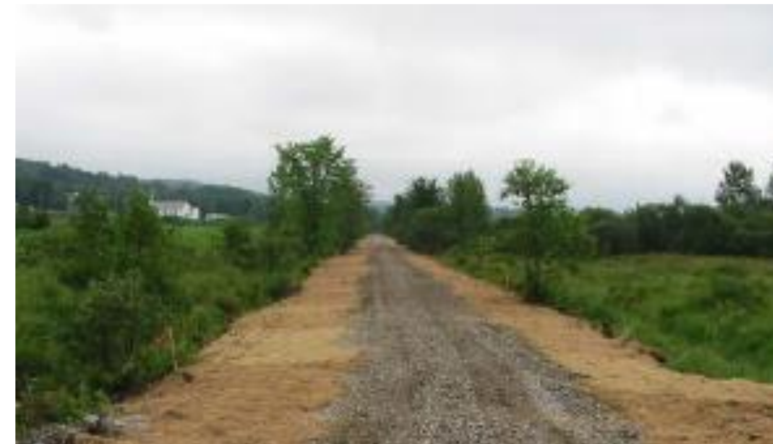
Figure 1. Example of rail bed lowered to the natural floodplain along Black Creek, Fairfield, VT.
