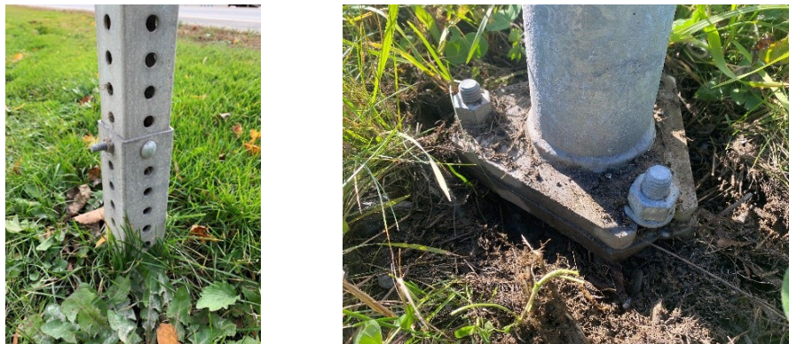
Figure 11. Breakaway devices applied in the field.
