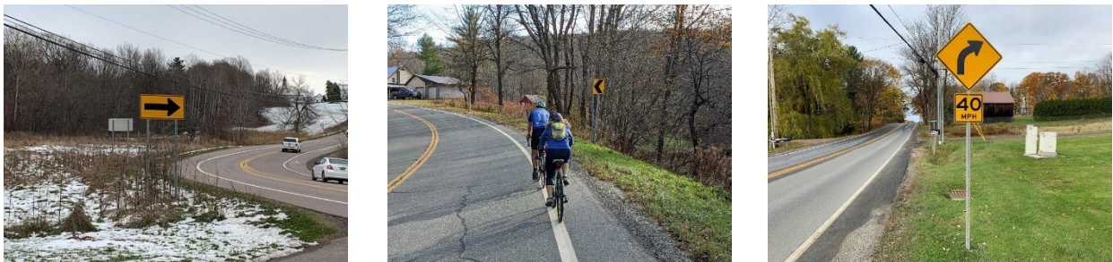
Figure 2. MUTCD Compliant Curve Warning Signs in Vermont.
