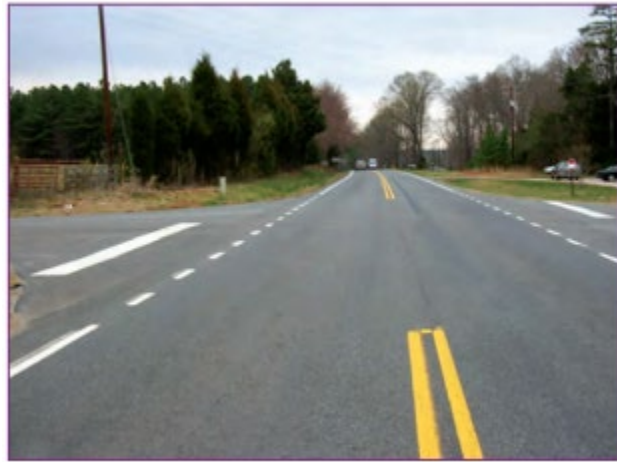
Figure 6. Application of pavement markings at intersections.
