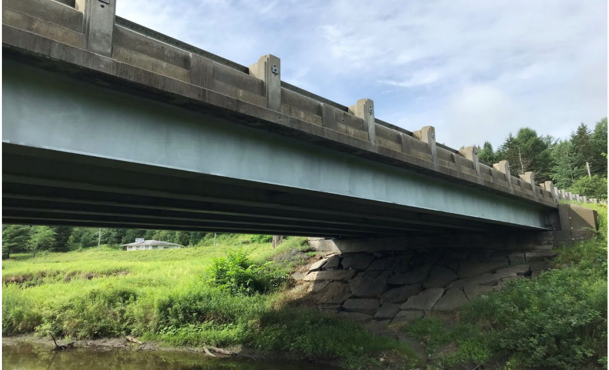
Finished Metalizing (Fascia Beam)
