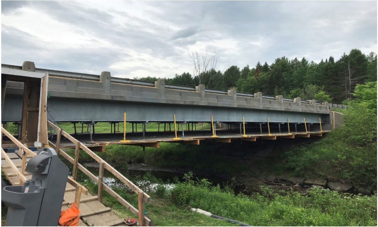
Work Platform Suspended from Beams
