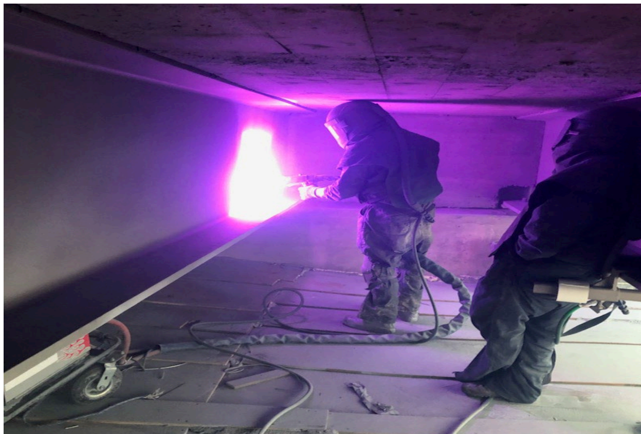
Metalizing Inside the Enclosure
