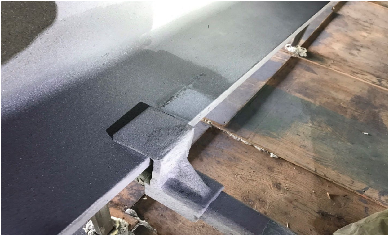
Repair Areas for Hanger Attachment
