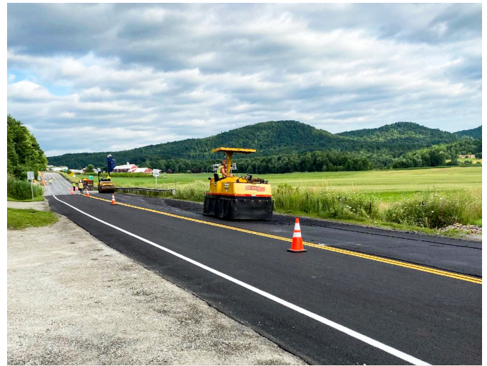
CAMBRIDGE. In 2020, VT-15 was resurfaced from the town of Underhill into Cambridge. This project used an asphalt recycling technique, saving on cost while providing a durable road surface.
