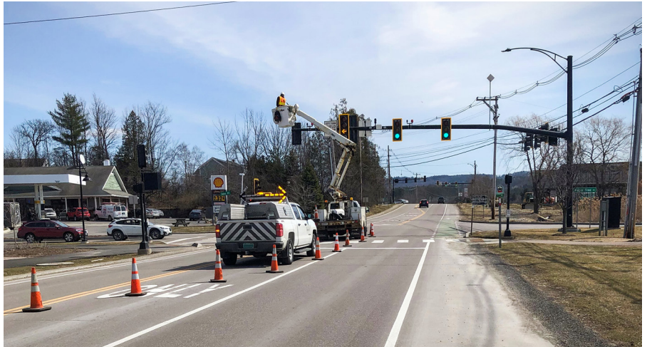
WILLISTON. The steep drop in traffic volumes early in the pandemic created some unique opportunities for different parts of the agency. Slower roadways allowed the VTrans Traffic Signal Unit to safely perform preventative maintenance at some of our busiest intersections.
