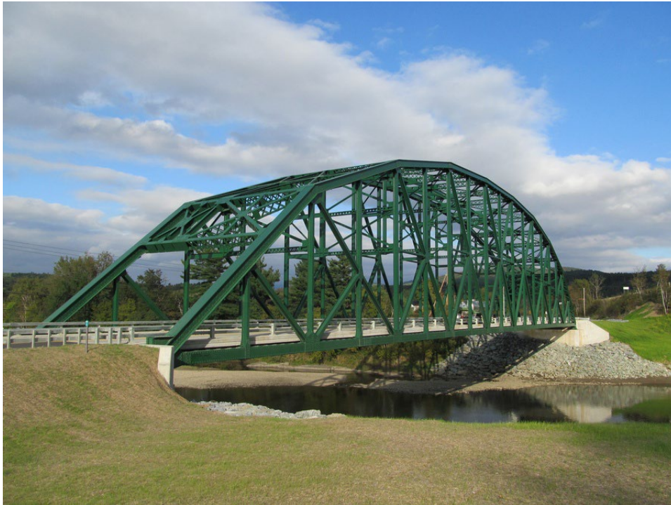
Checkered House Bridge Richmond VT
