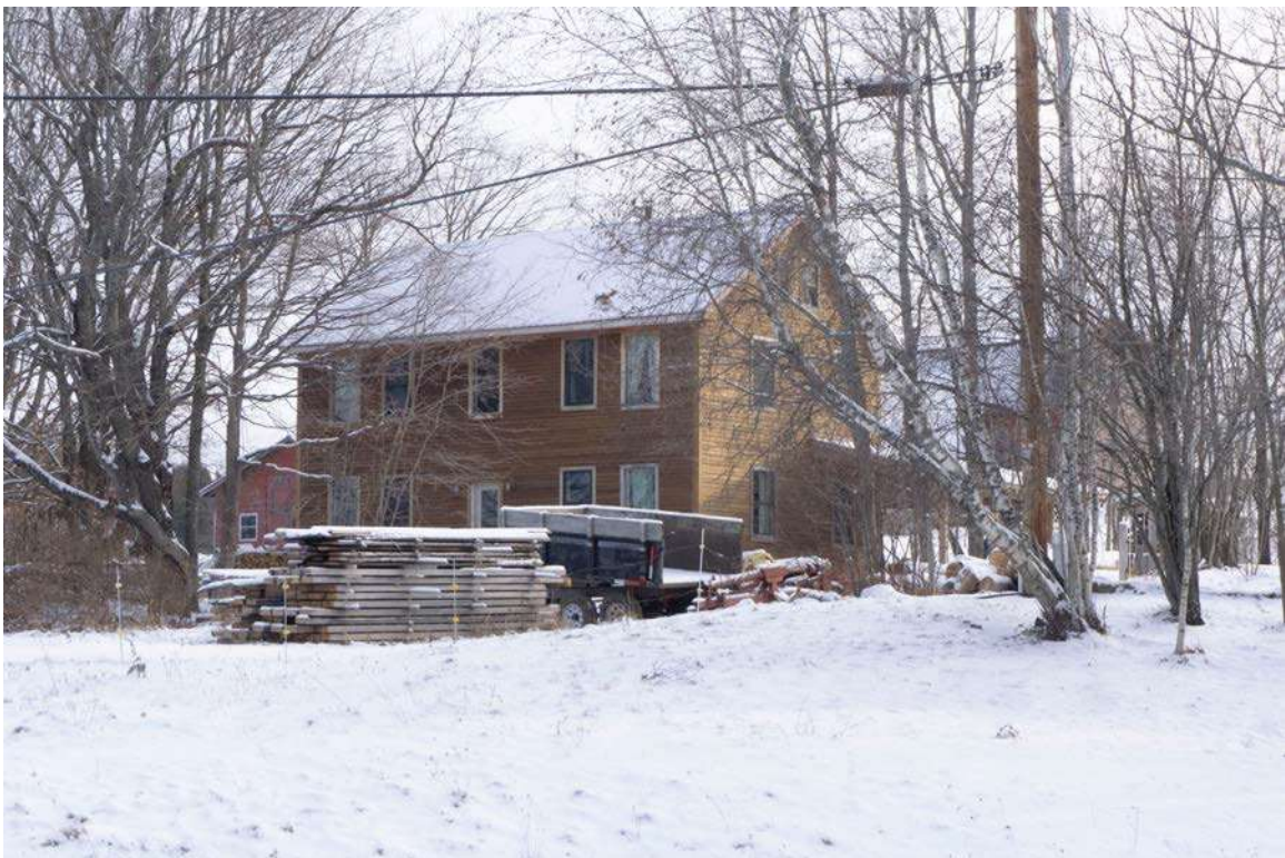
19. 1381 Airport Road looking southwest
