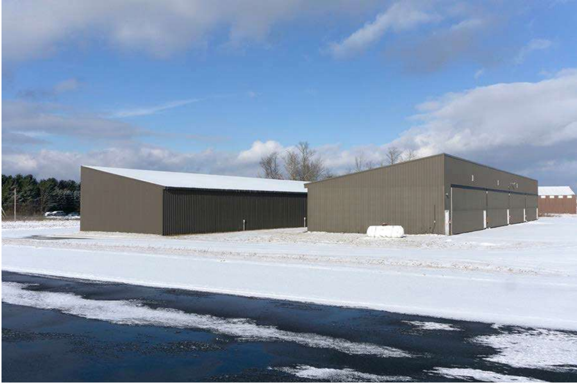
9. 1979 Airport Road looking northwest
