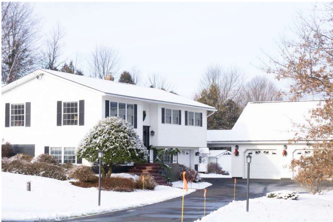
21. 1264 Airport Road looking northeast
