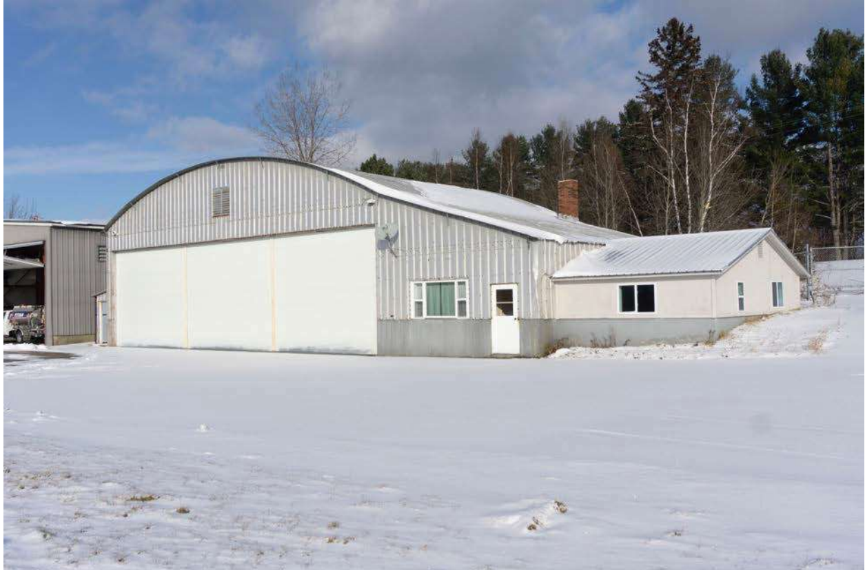
13. 1979 Airport Road, National Life hangar looking northeast
