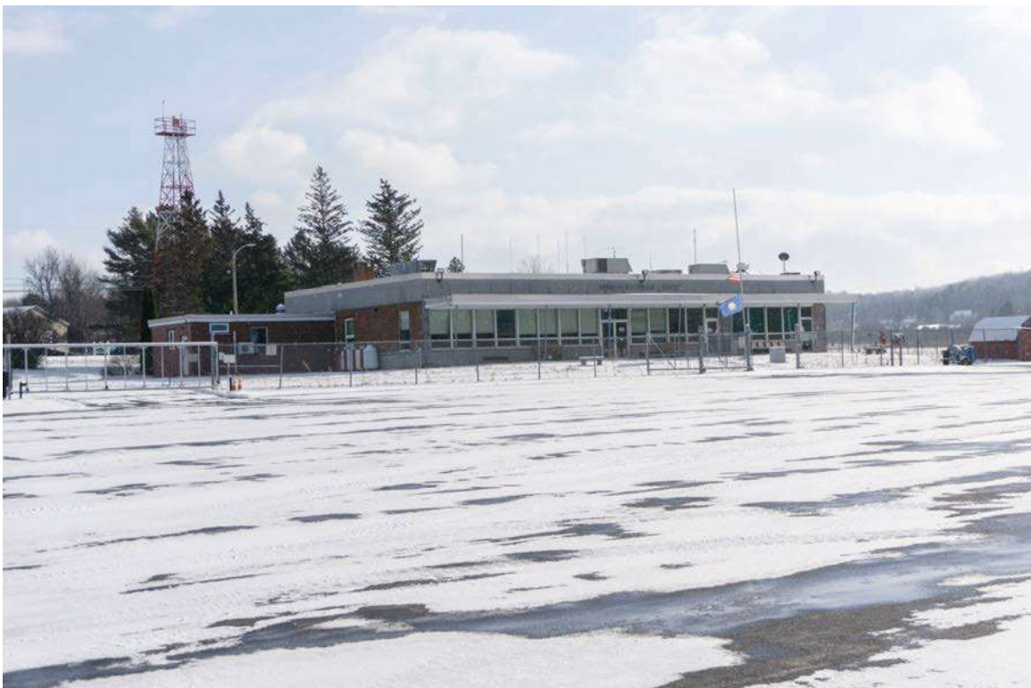
10. 1979 Airport Road, terminal looking south
