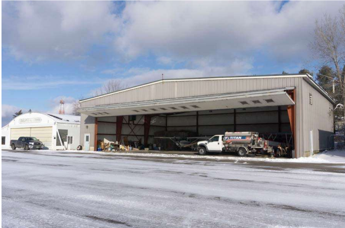
12. 1979 Airport Road, State Cold Storage looking northeast
