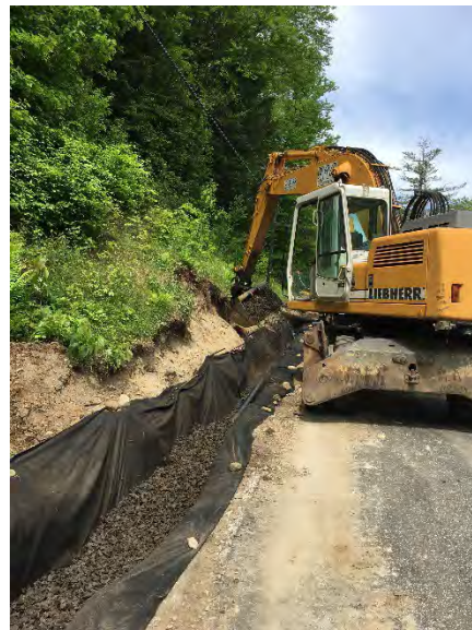
Placing TDA in fabric
