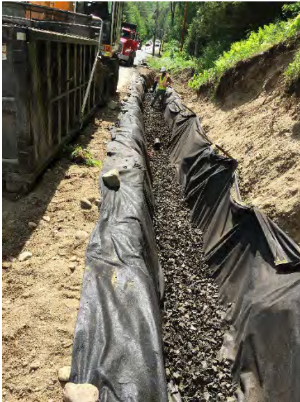
TDA placed over drainage pipe
