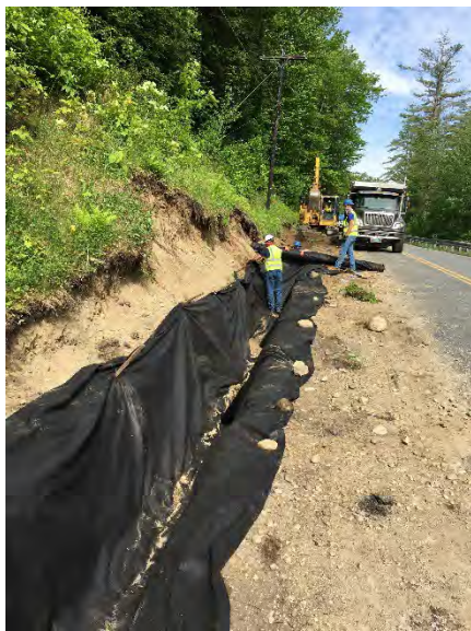
Fabric placed in trench
