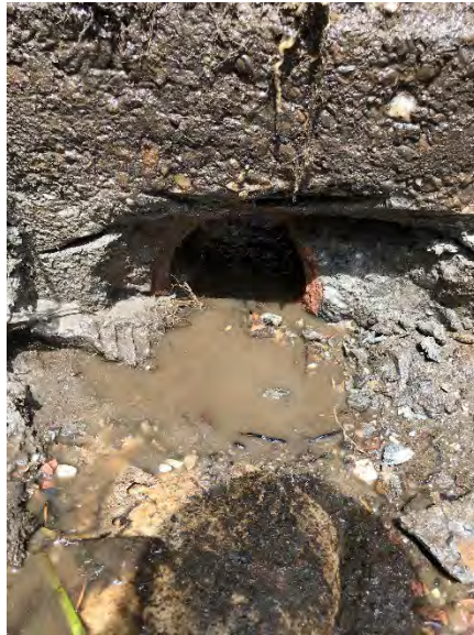
Figure 7: Drainage structure at Chester underdrain
