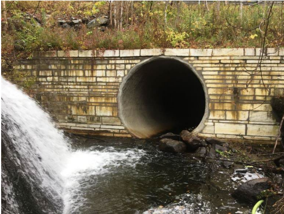
Figure 16. Weathersfield BR15 Spray On Liner: Inlet and headwall (2020)
