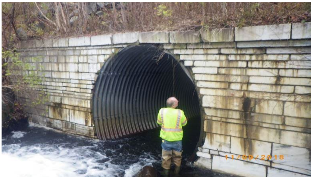
Figure 4. Weathersfield BR15 Inlet (2018 Inspection Photo)
