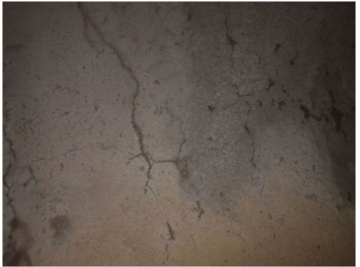
Figure(s) 23. Weathersfield BR15 Spray On Liner: side wall condition (left), minor cracking at culvert top (right) (2023)
