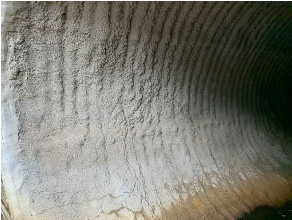
Figure 19. Weathersfield BR15 Spray On Liner: Spray-On pipe material near inlet (2021)
