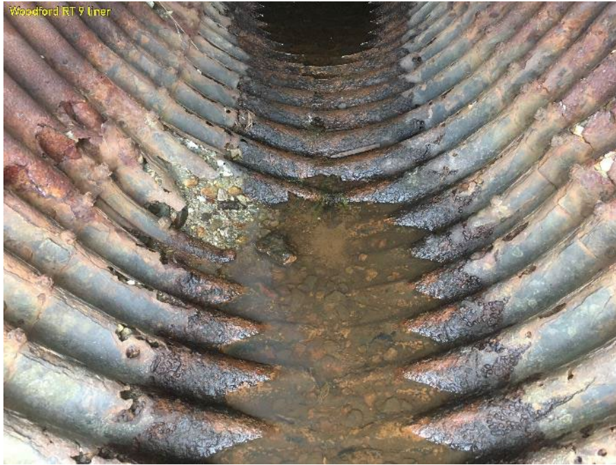
Figure 3. Woodford BR18 Invert Condition Pre-Spray on Liner Construction (Construction Photo)
