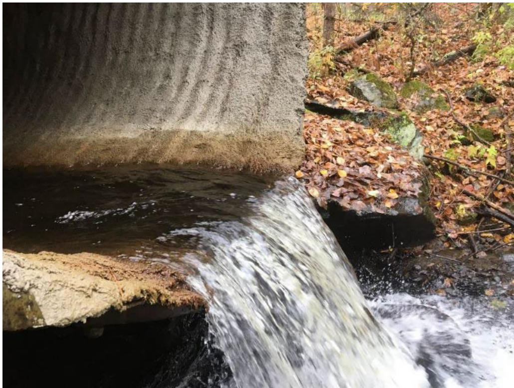
Figure 17. Weathersfield BR15 Spray On Liner: Outlet Invert (2020)
