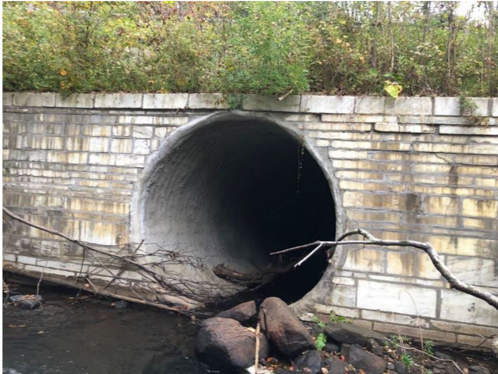
Figure 22. Weathersfield BR15 Spray On Liner: Inlet headwall (2023)
