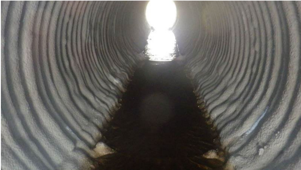
Figure 8. Woodford BR18 Spray On Liner: Barrel (2019)
