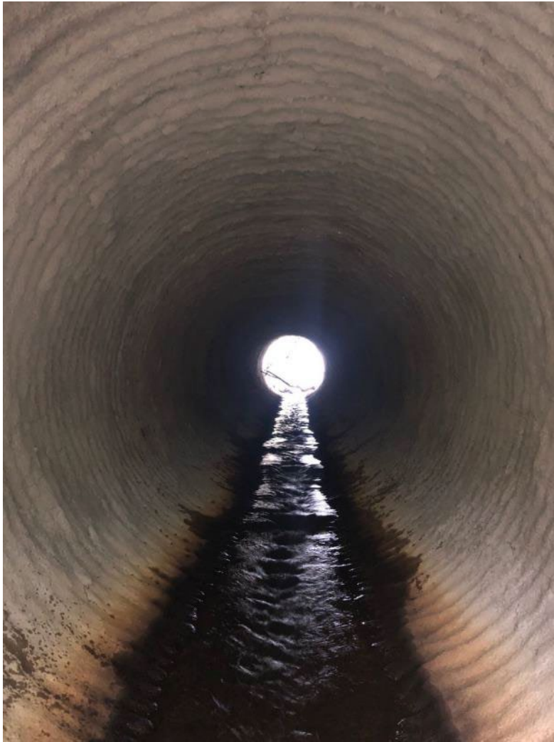
Figure 24. Weathersfield BR15 Spray On Liner: Barrel (2023)
