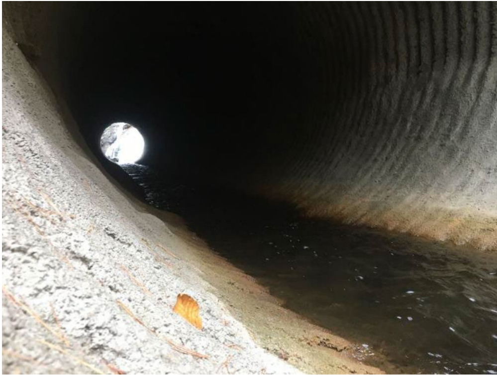
Figure 18. Weathersfield BR15 Spray On Liner: Invert minor staining (2020)
