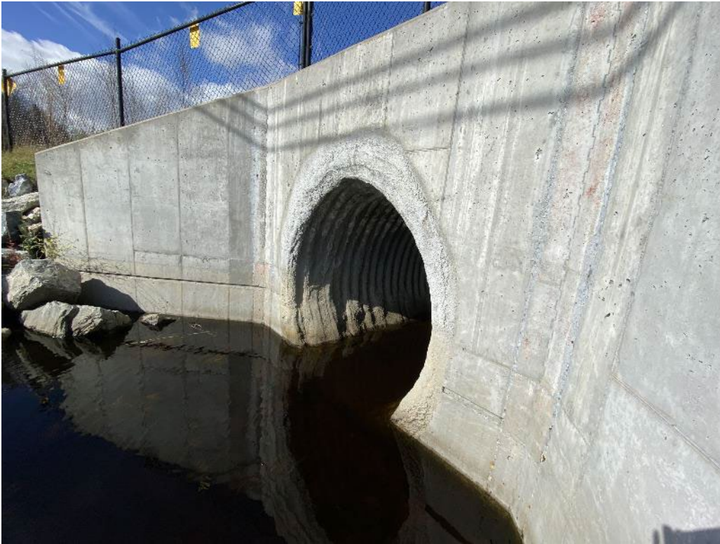
Figure 9. Woodford BR18 Spray On Liner: Inlet with beveled headwall (2021)
