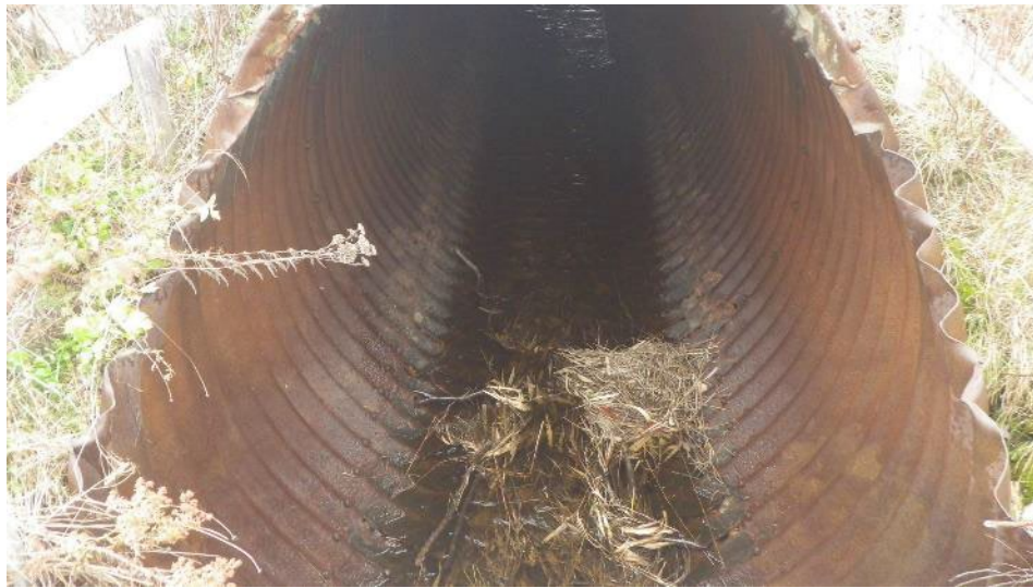
Figure 1. Woodford BR18 Inlet Invert (2016 Inspection Photo)
