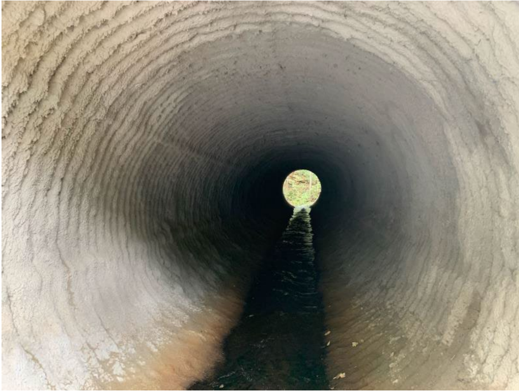
Figure 20. Weathersfield BR15 Spray On Liner: Barrel condition (2021)
