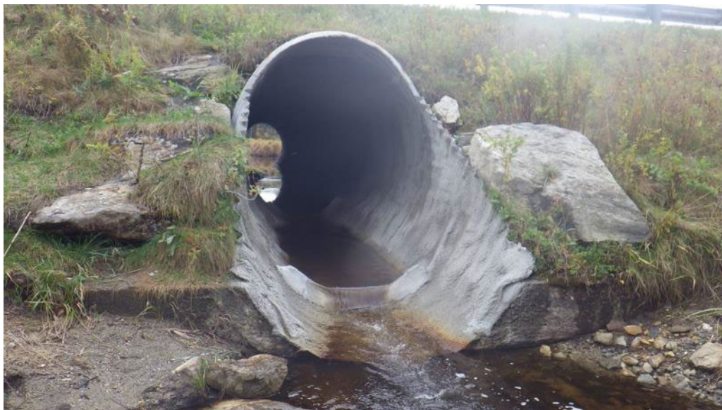
Figure 7. Woodford BR18 Spray On Liner: Outlet, fish baffles (2019)
