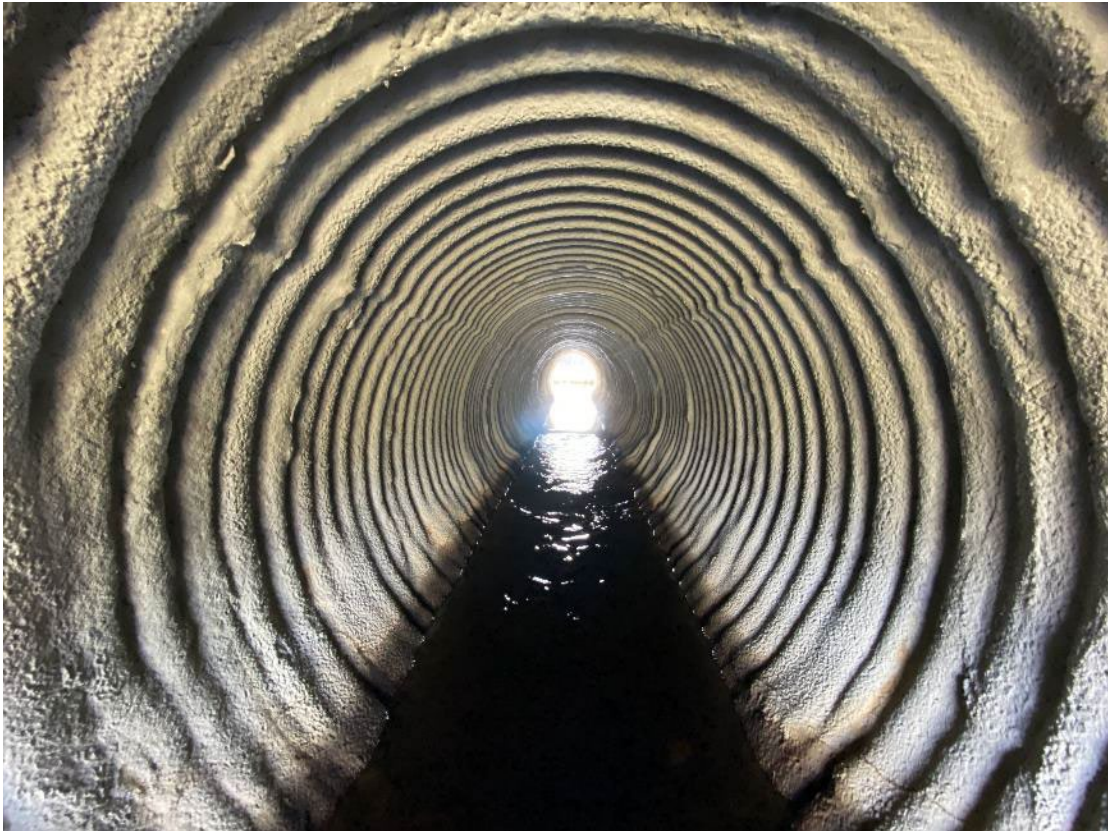
Figure 10. Woodford BR18 Spray On Liner: Barrel (2021)
