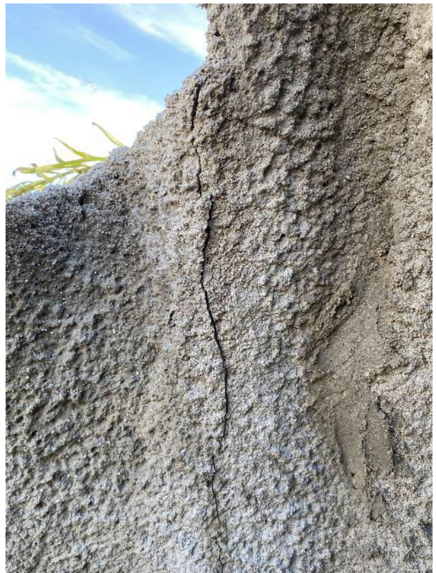
Figure 11. Woodford BR18 Spray On Liner: Staining along invert (left), Cracking along Outlet Mitered edge (right) (2021)
