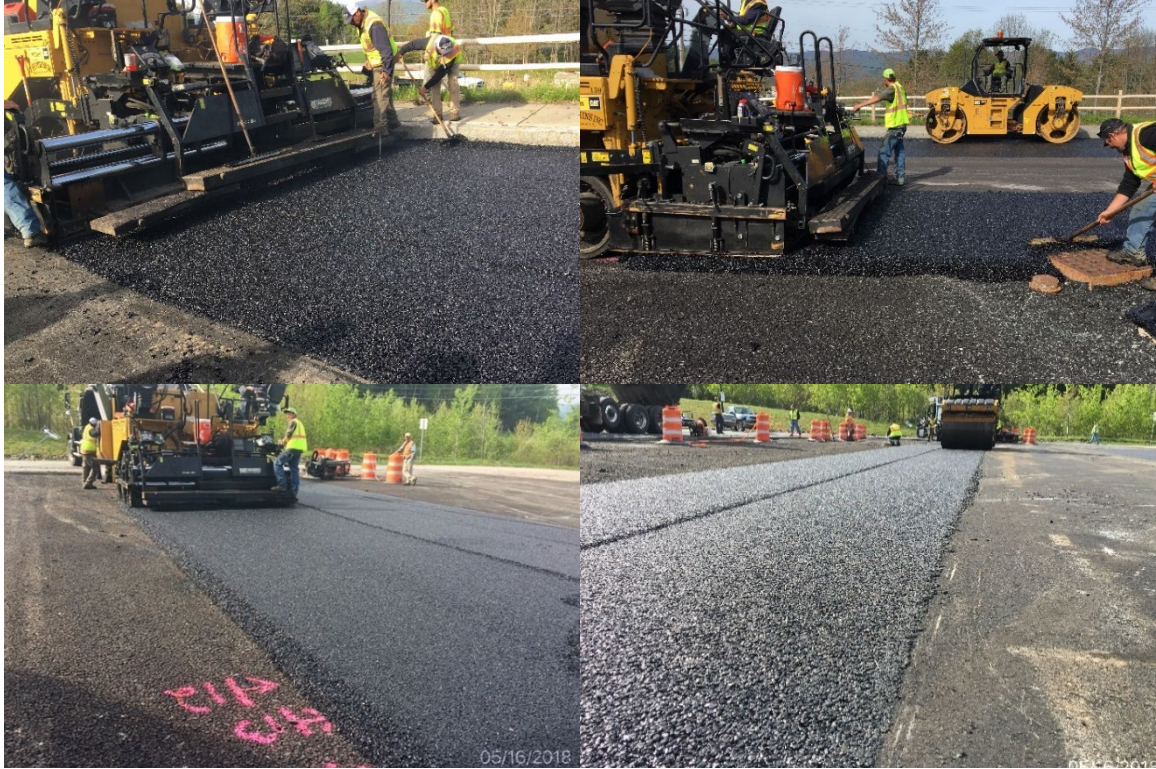
Figure 5: Open Graded Friction Course Paving
