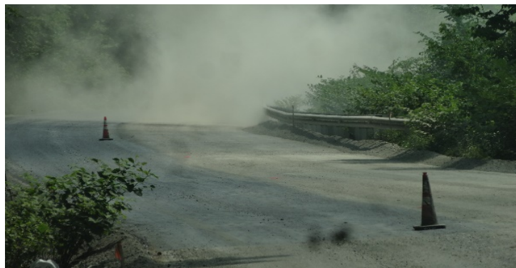
FIGURE 10. DUST PROBLEMS ON THE ROADWAY - PHOTO BY GCI
