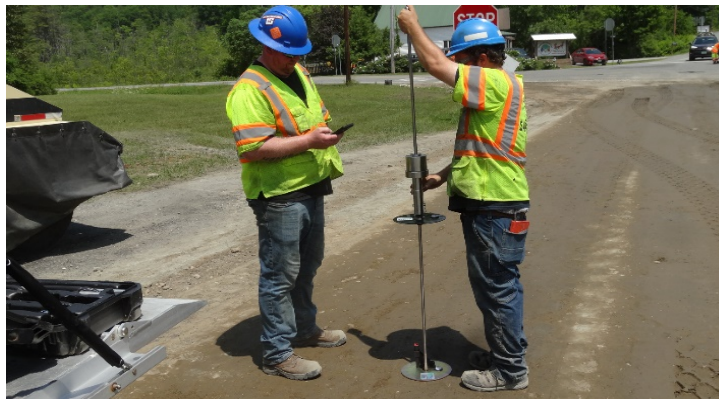
FIGURE 8. DCP TESTING - PHOTO BY GCI
