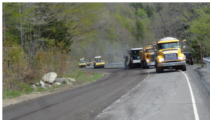
FIGURE 2. PULVERIZATION OPERATIONS - PHOTO BY GCI
