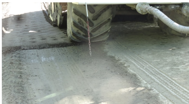
FIGURE 4. OVERLAPPING OF RECLAMATION PASSES - PHOTO BY GCI
