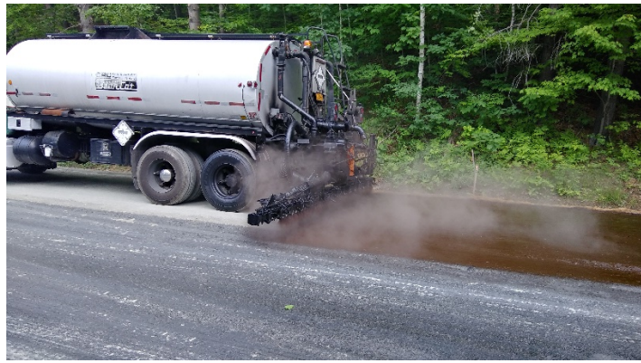
FIGURE 11 EMULSION SEAL COAT BEING APPLIED - PHOTO BY GCI
