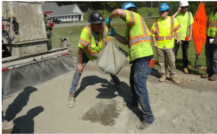
FIGURE 6. CEMENT CANVAS PATCH TEST - PHOTO BY GCI
