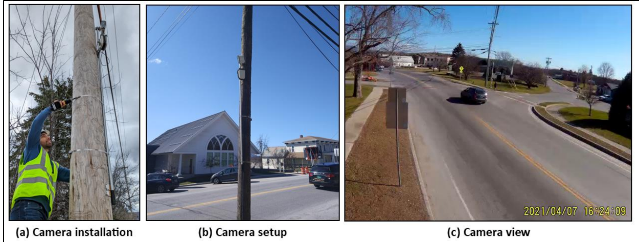
Figure 5: CountCam installation and use at the RRFB treatment location in Middlebury.
