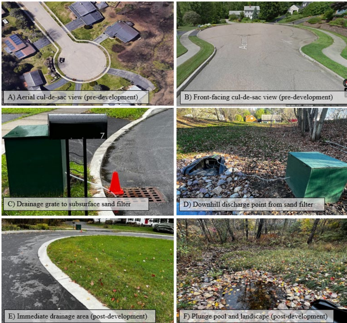
Figure A2. The pre and post development progress of Site A. A) Aerial cul-de-sac view (pre-development) is an arial image of the cul-de-sac branching from the neighborhood. B) Front-facing cul-de-sac view (pre-development) is the front-facing view to the end of the cul-de-sac before the sand filter was constructed. C) Drainage grate to subsurface sand filter shows the point from which runoff exits the landscape and enters the treatment system. D) Down-hill discharge point from sand filter shows the point from which treated water exits the system. E) Immediate drainage area (post-development) shows the immediate drainage area with the entry point in C) visible in the top center of the image. This grassed area was not in B). F) Plunge pool and landscape (post-development) shows the plunge pool and immediate drainage area into a wooded landscape. Images A and B were obtained from Google Earth. Images C-F were taken by M. Schambura.
