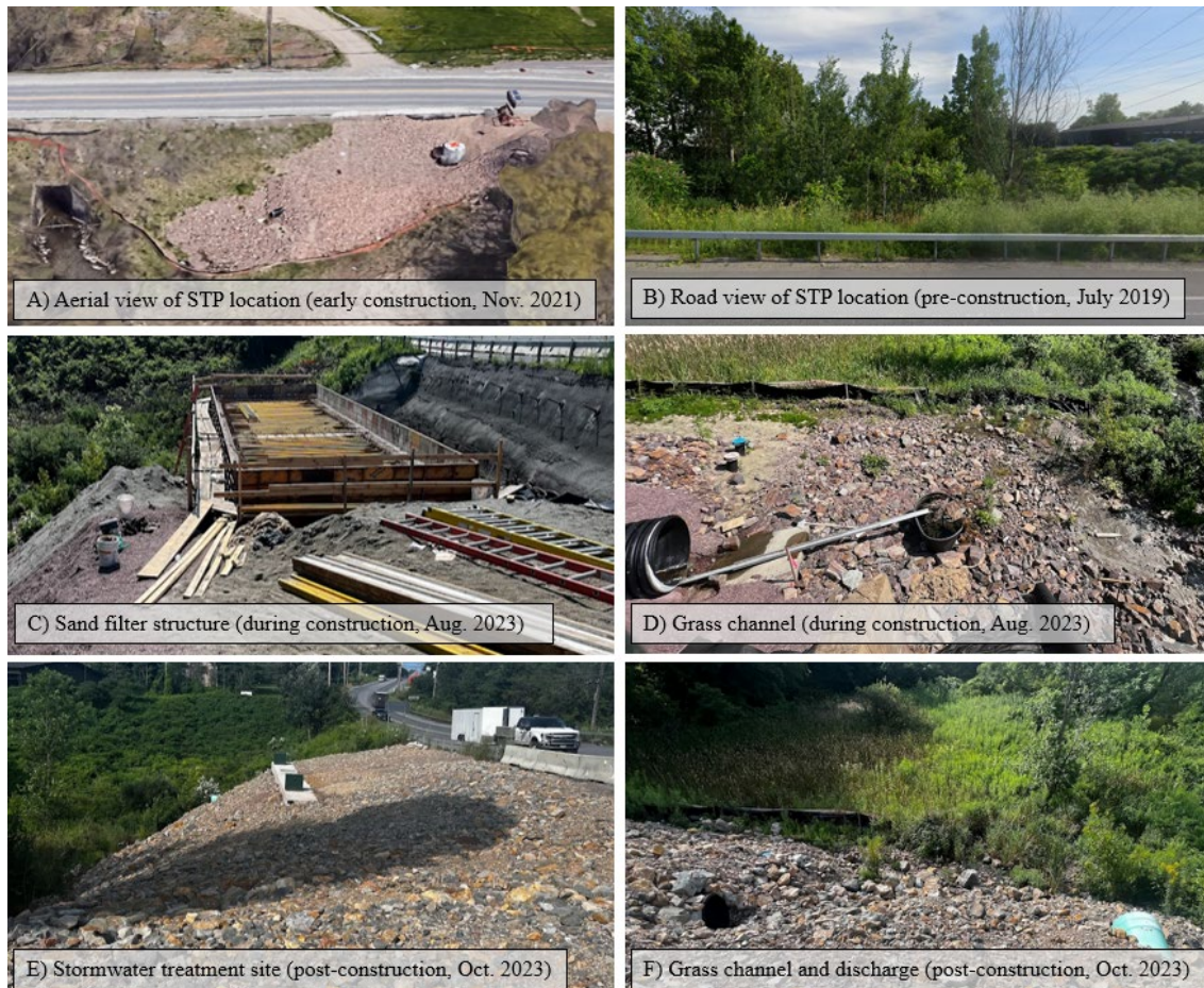
Fig A3. The pre and post development progress of Site B. A) Aerial view of STP location (early construction, Nov. 2021) shows the location for the sand filter and stone-lined slope after the project began. The Muddy Brook River is shown in the bottom left corner. B) Road view of STP location (pre-construction, July 2019) shows the view before construction began. C) Sand filter structure (during construction, Aug. 2023) shows the frame of the sand filter next to U.S Route 2. D) Stone-lined slope and vegetated riparian area (during construction, Aug. 2023) shows the treatment area, pre-seeded. E) Stormwater treatment site (post-construction, Oct 2023) shows the finished site with boxes for monitoring equipment atop the surface. F) Stone-lined slope that drains to a vegetated riparian area (post-construction, Oct 2023). Runoff exclusively conveyed by the stone-lined slope is discharged from the black pipe (left), and runoff treated by the sand filter during high flows is discharged from the blue pipe (right) and conveyed to the stone-lined slope/vegetated riparian area. Image A was obtained from Google Earth. Image B was obtained from Google Maps History. Images C-F were taken by M. Schambura.
