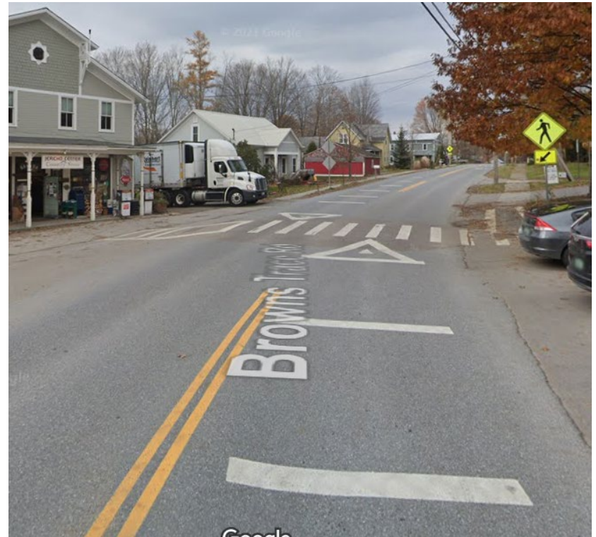
Raised crosswalk in Jericho Center, Vermont
