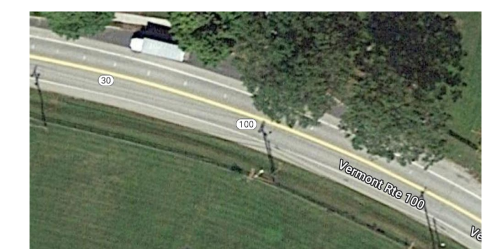
Figure 8. Remains of transverse line markings in Jamaica, Vermont
