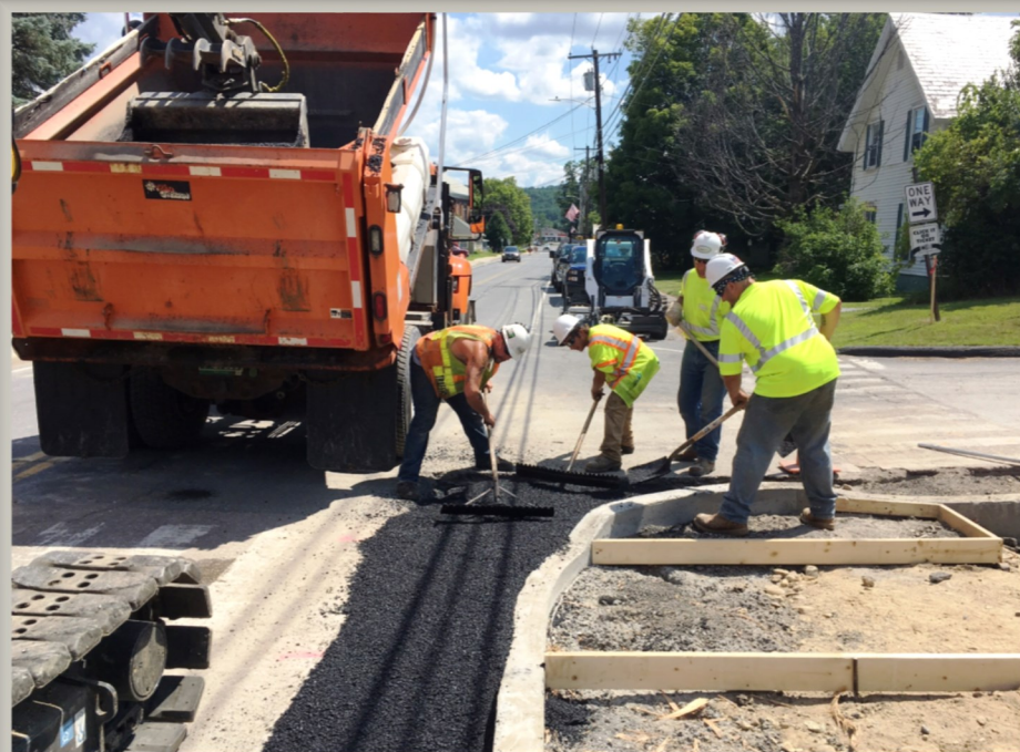
Castleton Crew installing Safe Routes to Crosswalk in West Rutland
