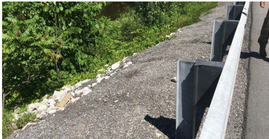
Erosion Fix, US Route 4 in Proctor, VT
