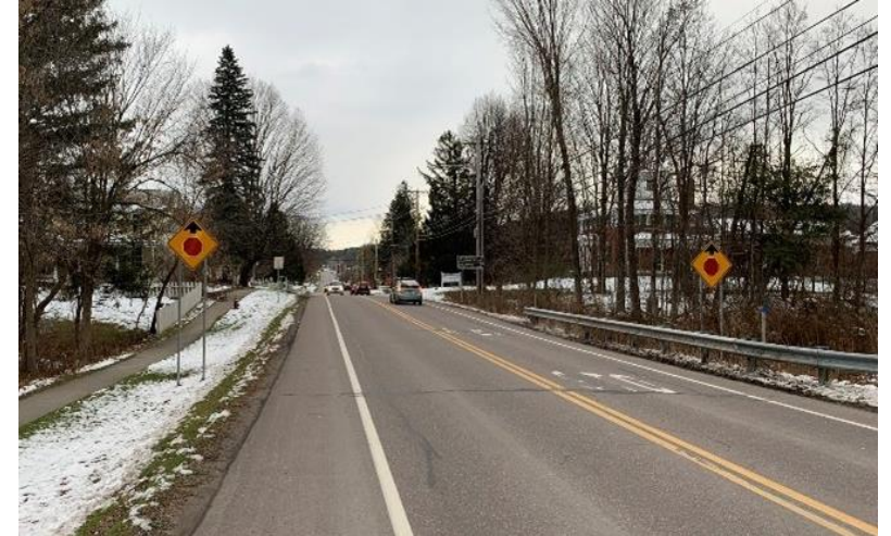
Figure 5. Application of intersection signage in Vermont.
